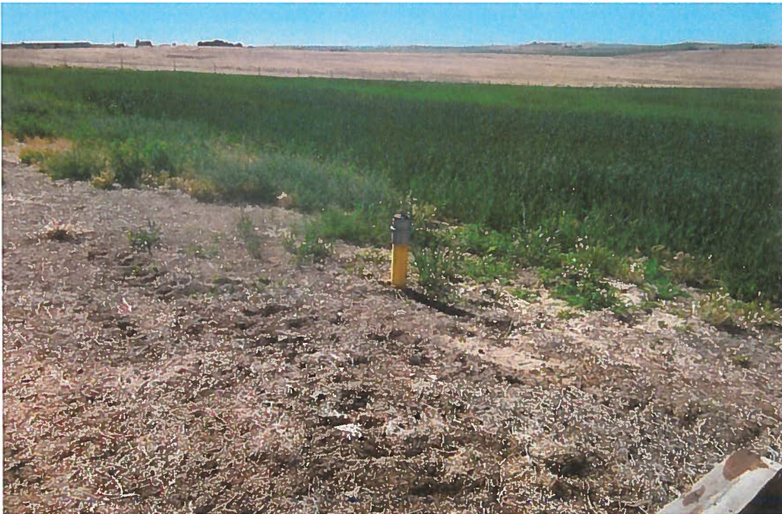
One of the 13 risers.
