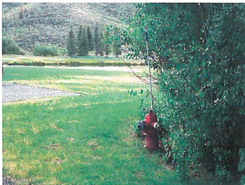
Figure 4: Hydrant at northwest corner of pond.
