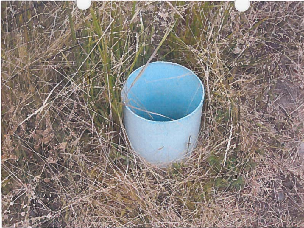
PVC control valve box. Each spring and each trough has a control valve.
