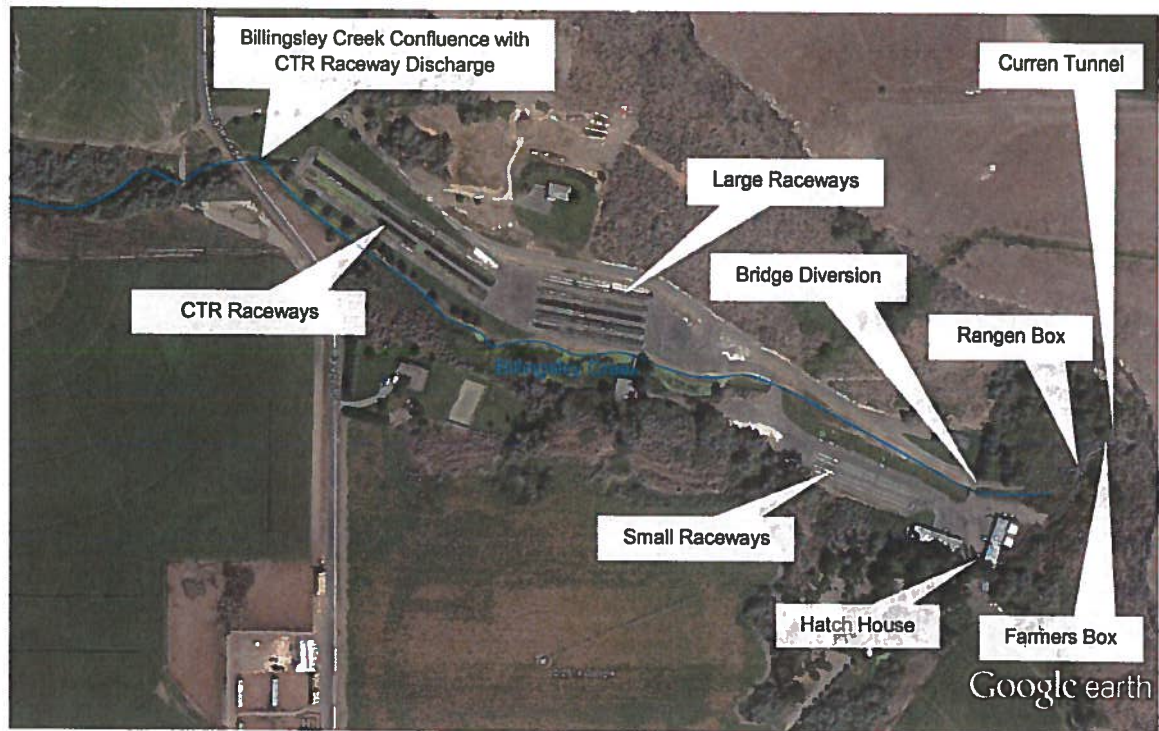
Figure 1. Aerial Photo of Major Water Supply Features for Rangen Aquatic Research Center
