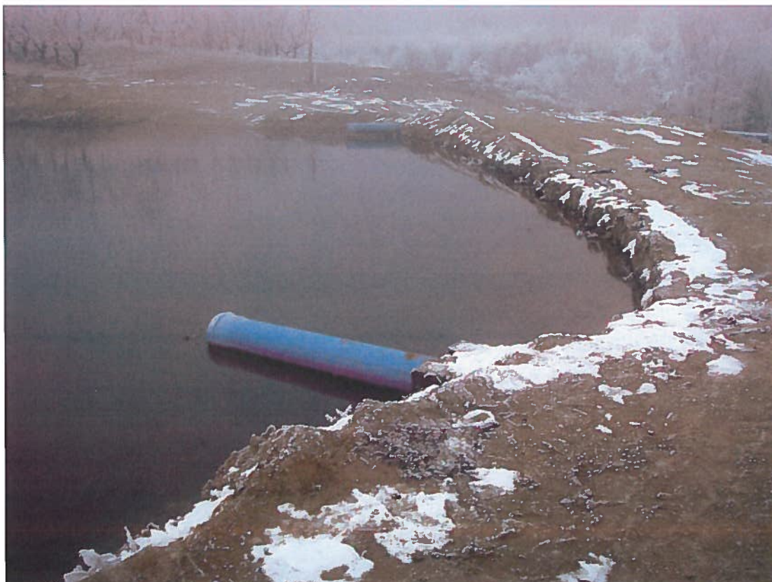
Photo No. 2, looking at dam crest from right abutment.
