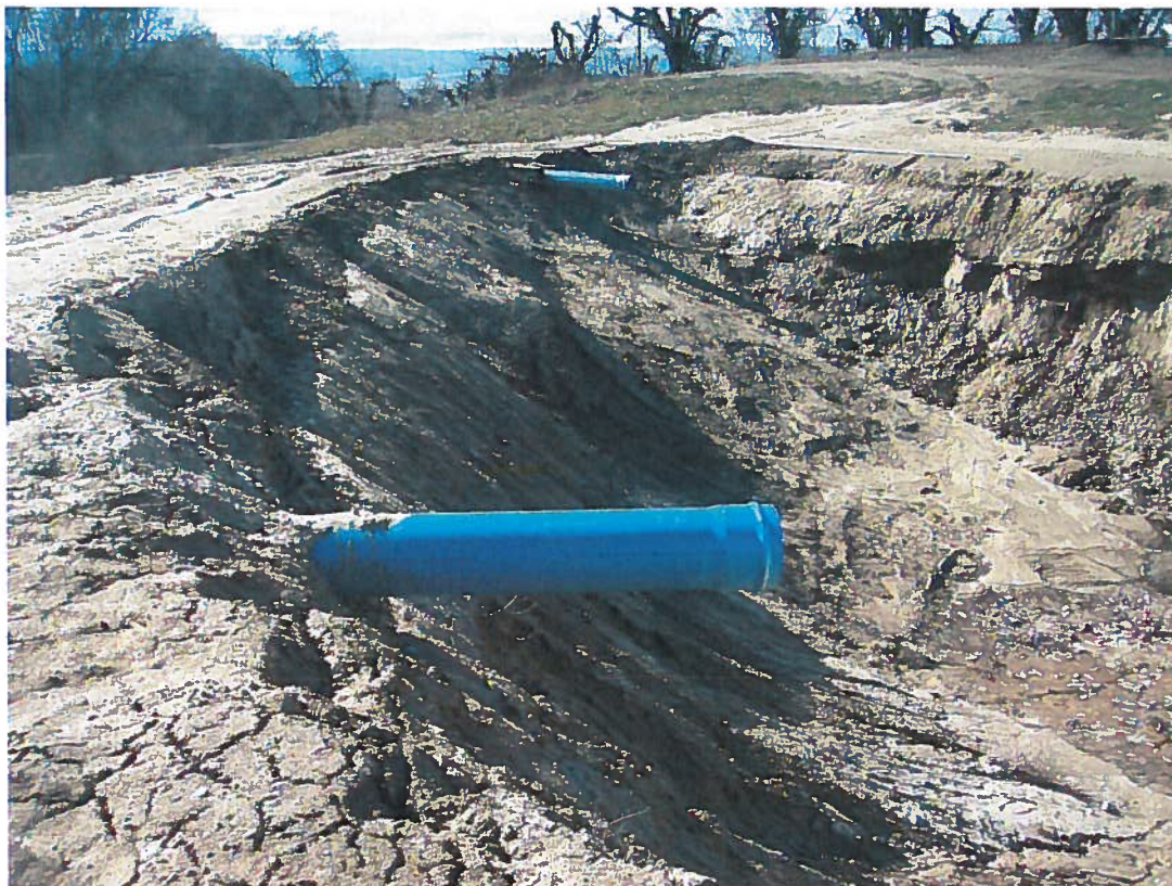
Photo No. 3, viewing embankment upstream slope from left abutment showing outlet pipes position.
