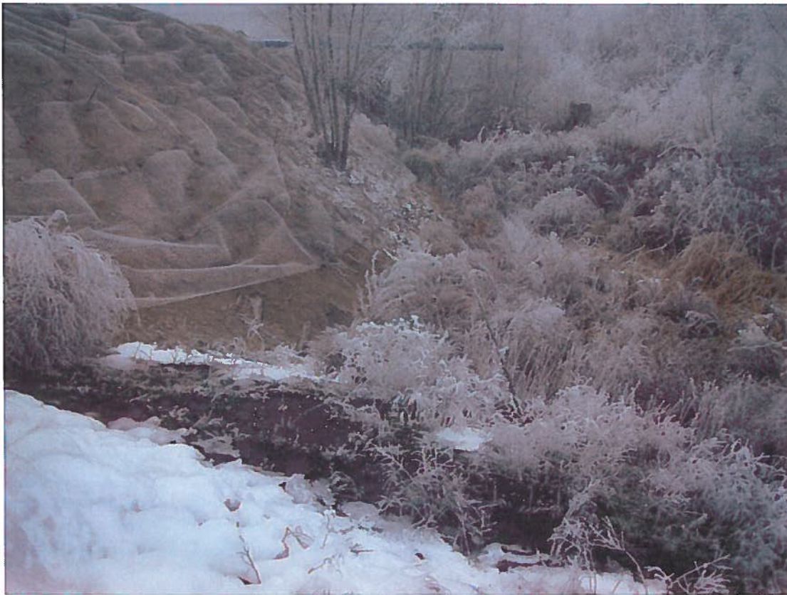
Photo No. 12 viewing downstream face of embankment looking toe area and tree on downstream face of dam.
