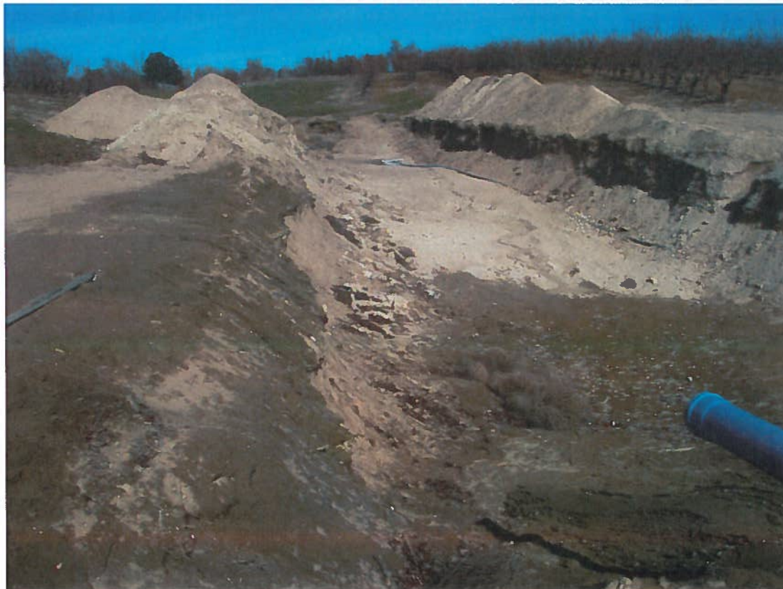
Photo No. 2, viewing impoundment excavation from right abutment.
