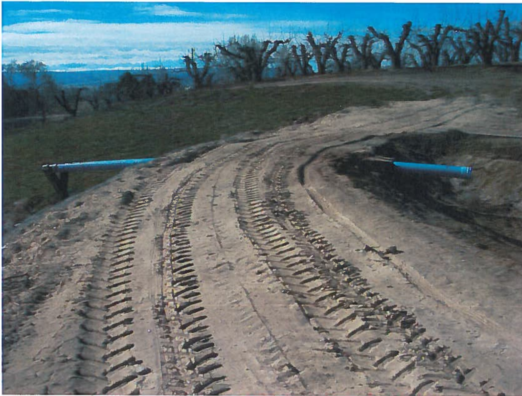
Photo No. 5, viewing dam crest from left side of dam showing newly placed material to level crest and provide access to orchards.
