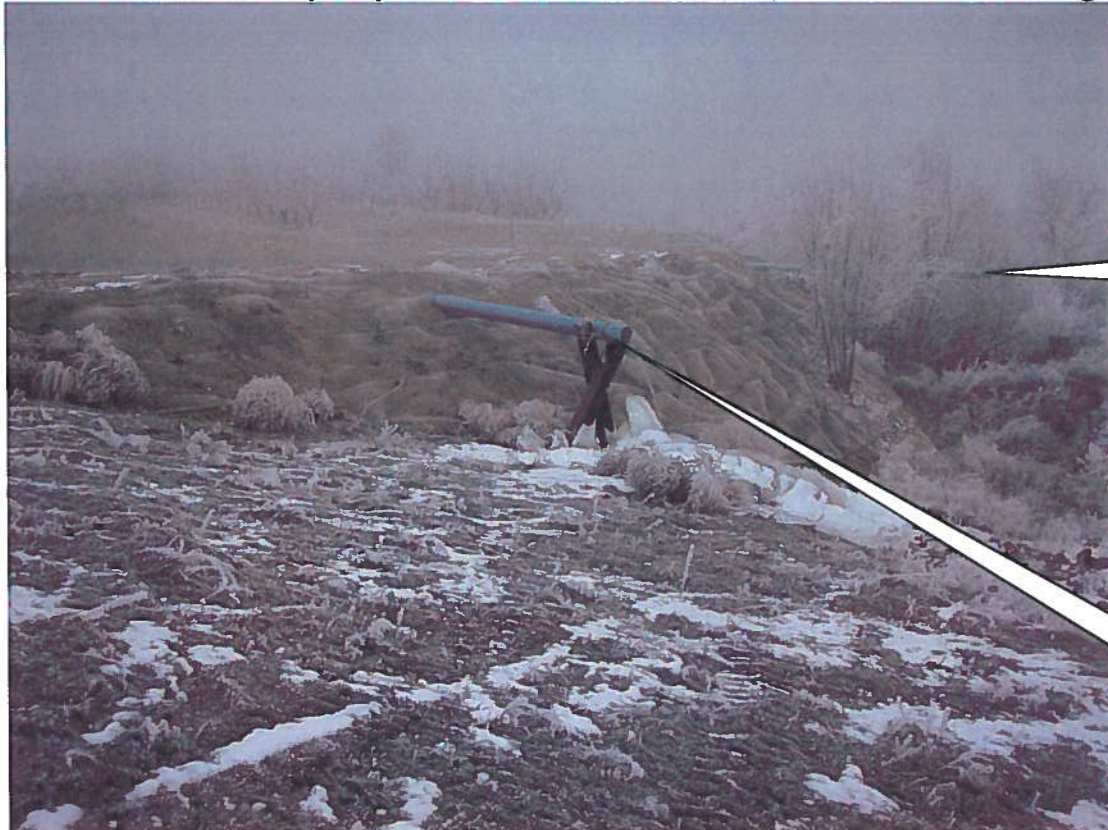
Photo No.1 viewing embankment from point downstream of right abutment.
