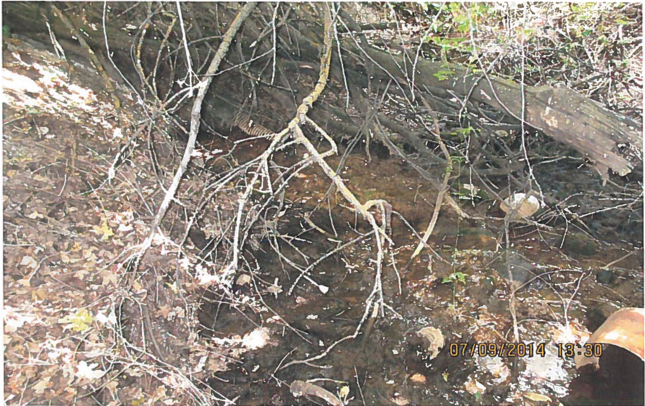
Photo # 1 -112.425957, 42.823617.. Looking SW.. Not sure what this is... water and brown sludge flowing in surrounding the pipe and lots of algae growth downstream. Suspect it is a toilet drain, didn't see any paper and didn't want to get to close.
