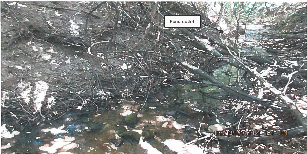
Photo # 2 looking NE, downstream algae growth from the pipe, the pond outlet is indicated in the photo..
