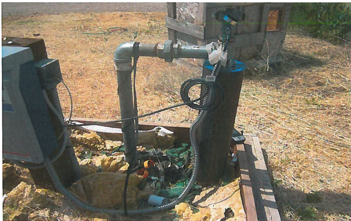
POD – Well with submersible pump. Steel pipe from well conveys water to buried 2 inch PVC pipe to 6000 gallon storage tank in shed. Storage tank seen in photograph below.
