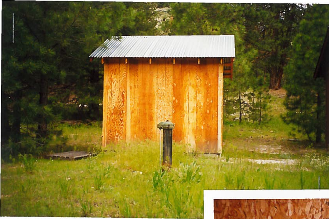
① Well, behind pump shed
