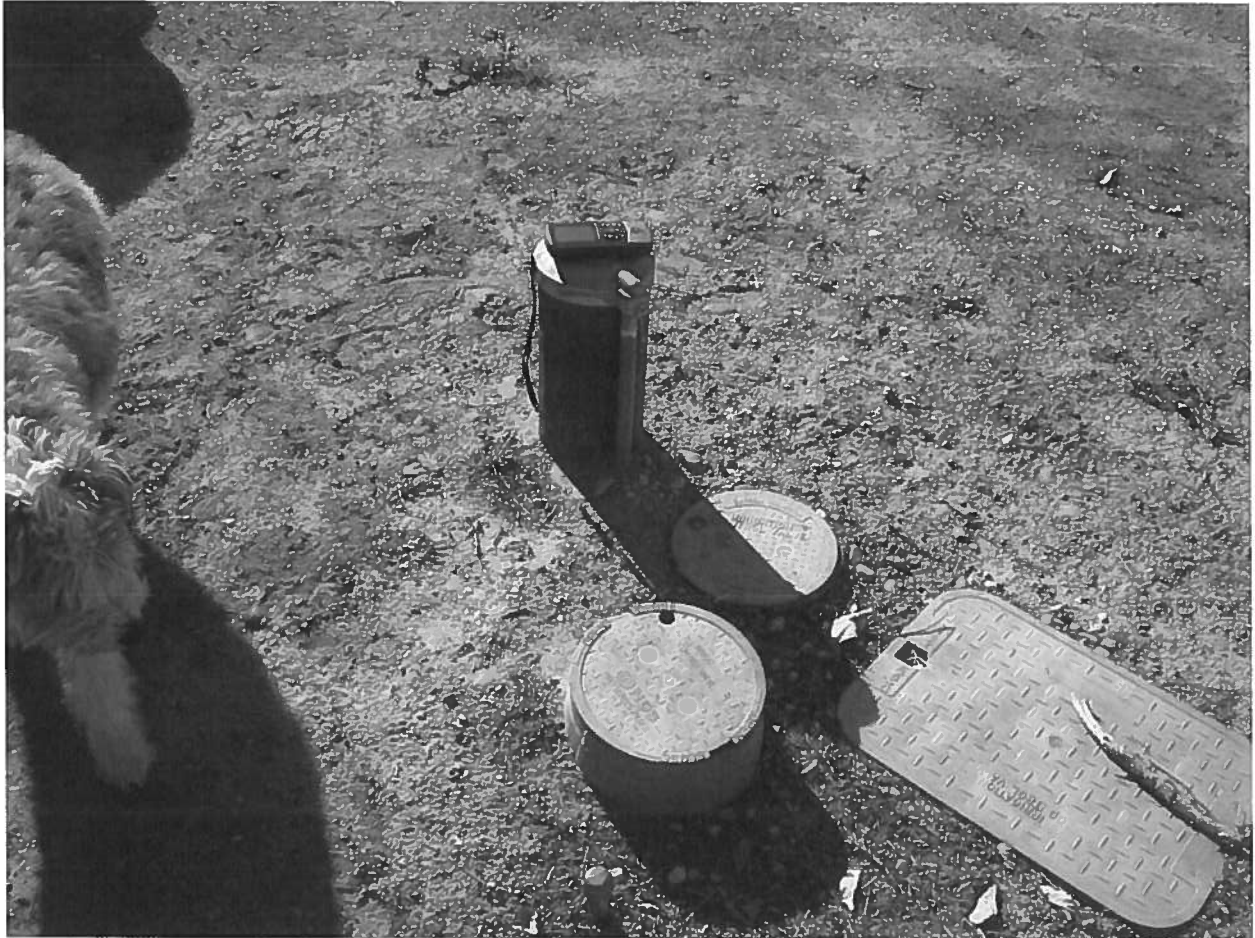
63-31753 Exam 10/24/2013: POD well with irrigation control valve box.
