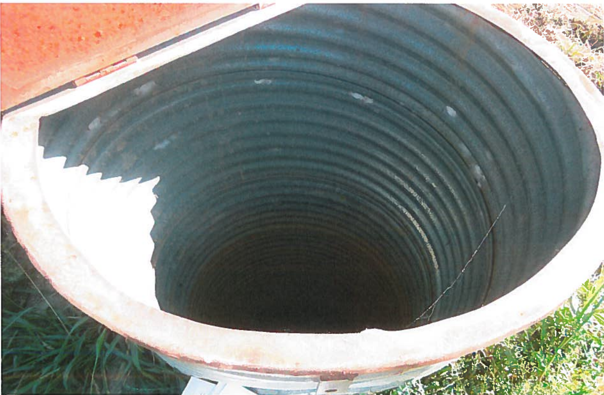
Both photographs on this page are views of the 24 –inch diameter, 17-foot deep “shallow well”
