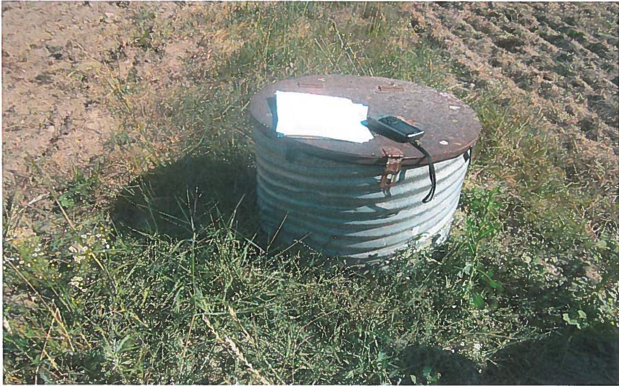
Both photographs on this page are views of the 24 –inch diameter, 17-foot deep “shallow well”
