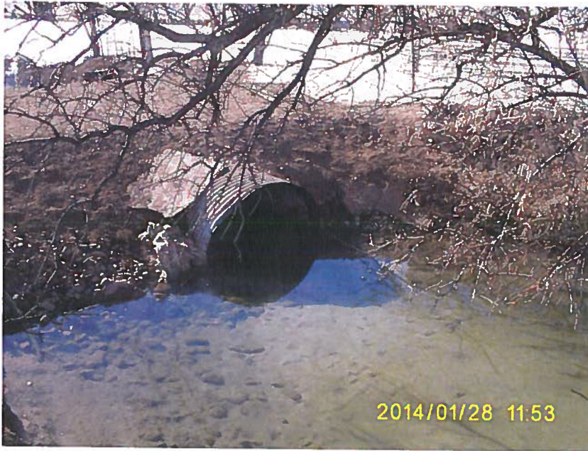
Photo 7739. Outlet culvert from Warm Springs. Note plywood boards. Note the fine silty-appearing material in channel center.
