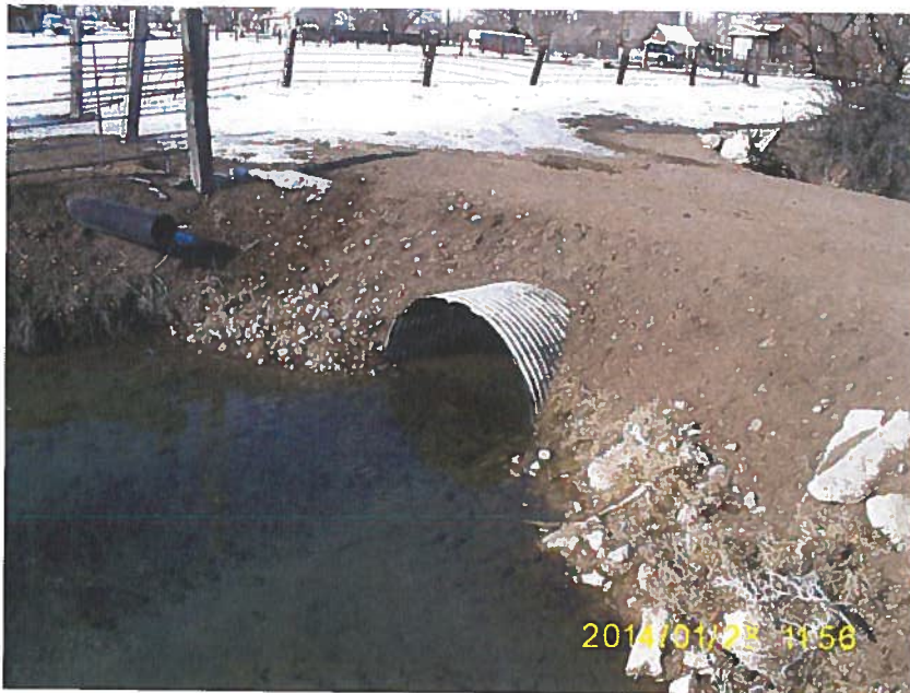
Photo 7740. Exit point of outlet culvert. Velocity-head rod measurements were made at this point.
