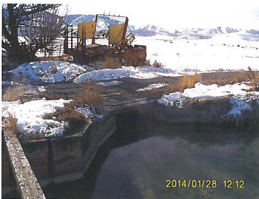
Photo 7746. Concrete outlet channel from junction box.
