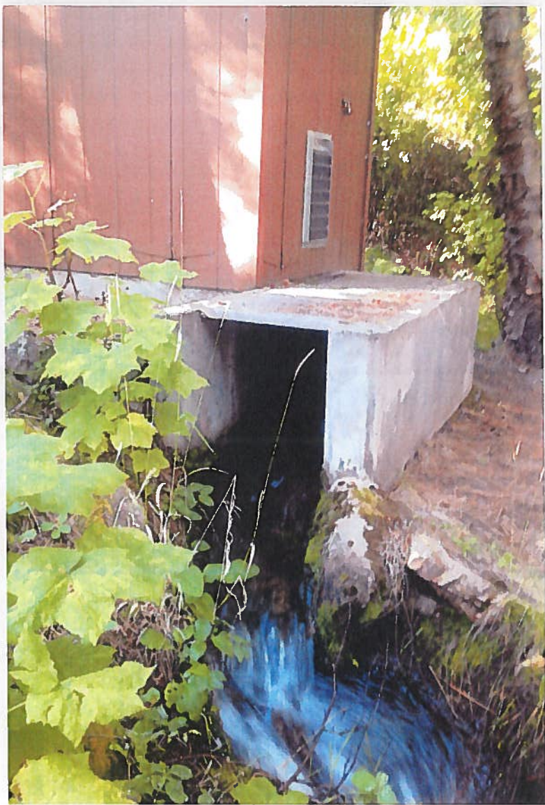
View of the Power House. concrete Raceway. Water is discharged to an open ditch which discharges water to a settling pond.
