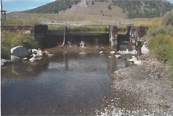
Photo 1: Existing diversion structure, August, 2004
