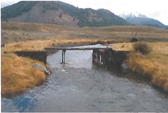
Photo 7: Existing diversion with boards pulled, October, 2001
