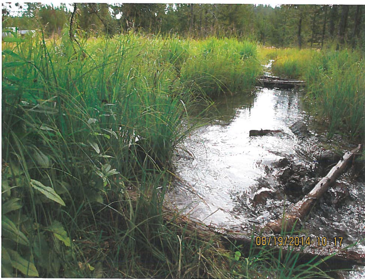
Return pipe in channel
