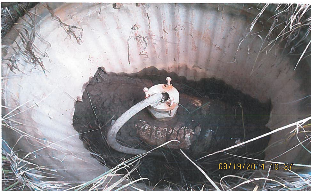
Measuring port in pipe near headgate
