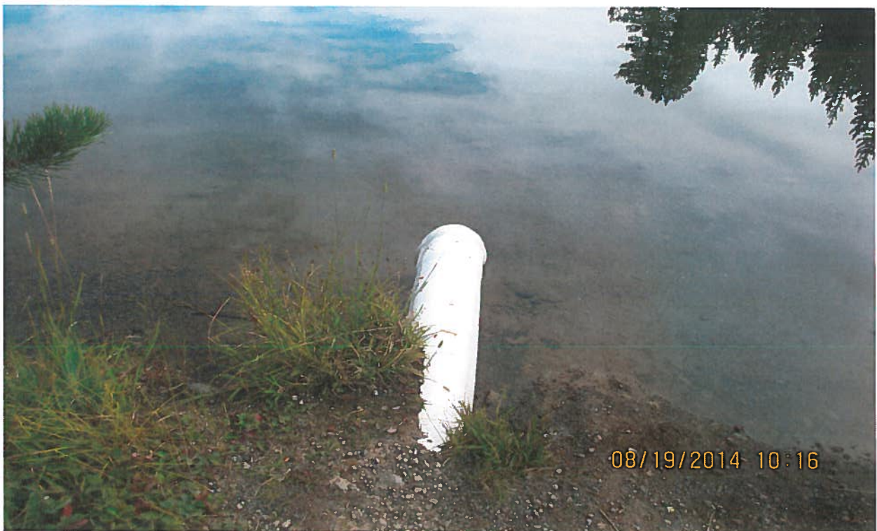
Outflow pipe from lake, looking North
