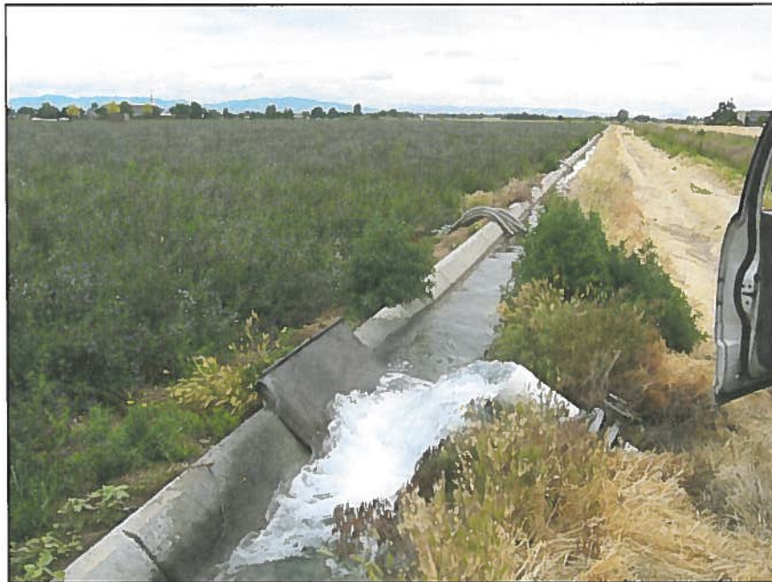
Figure 12: Well #2 discharge pipe to concrete ditch. Photo facing east.
