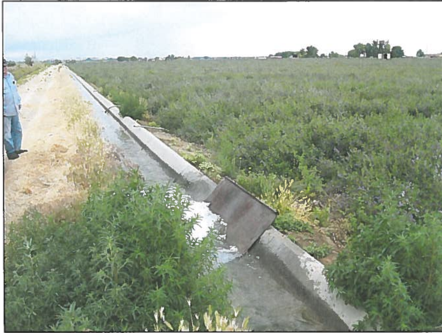
Figure 11: Well #2 discharge to concrete ditch. Photo facing west.
