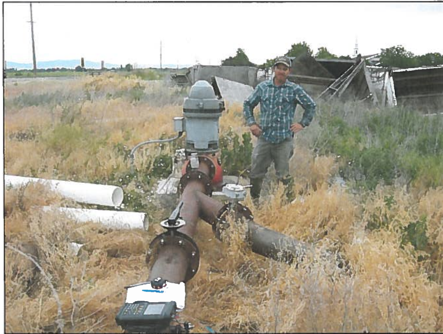
Figure 1: Well #1 facing easterly. Pipeline on right conveys flow to south end of farm and the near pipeline conveys flow across Kuna Road to the north.
