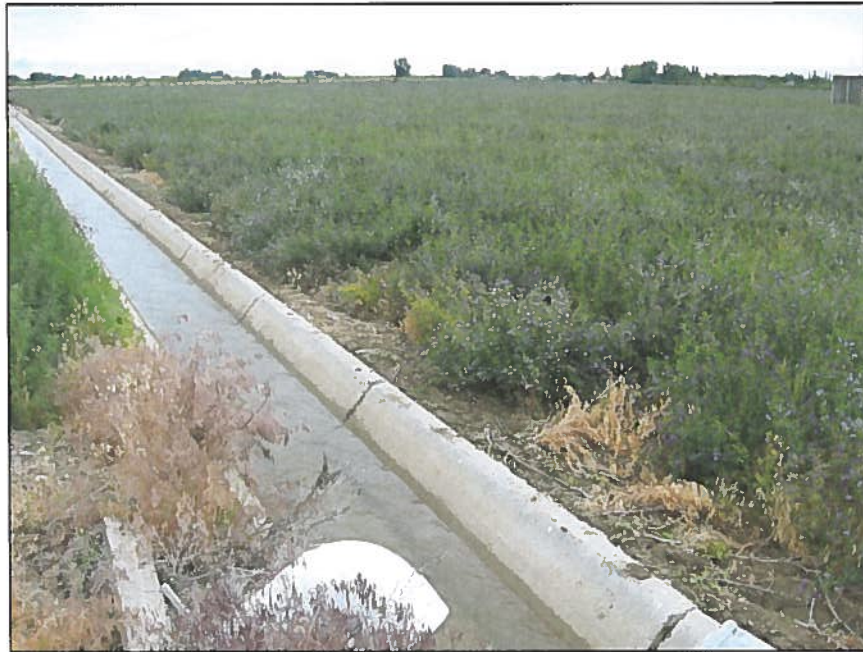
Figure 5: Northeast discharge point facing northerly showing place of use.
