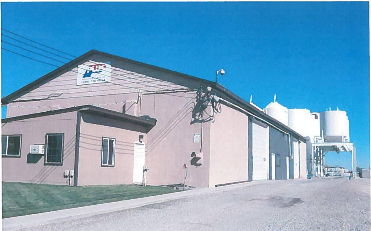
Below: Manufacturing facility with a break room and restrooms
