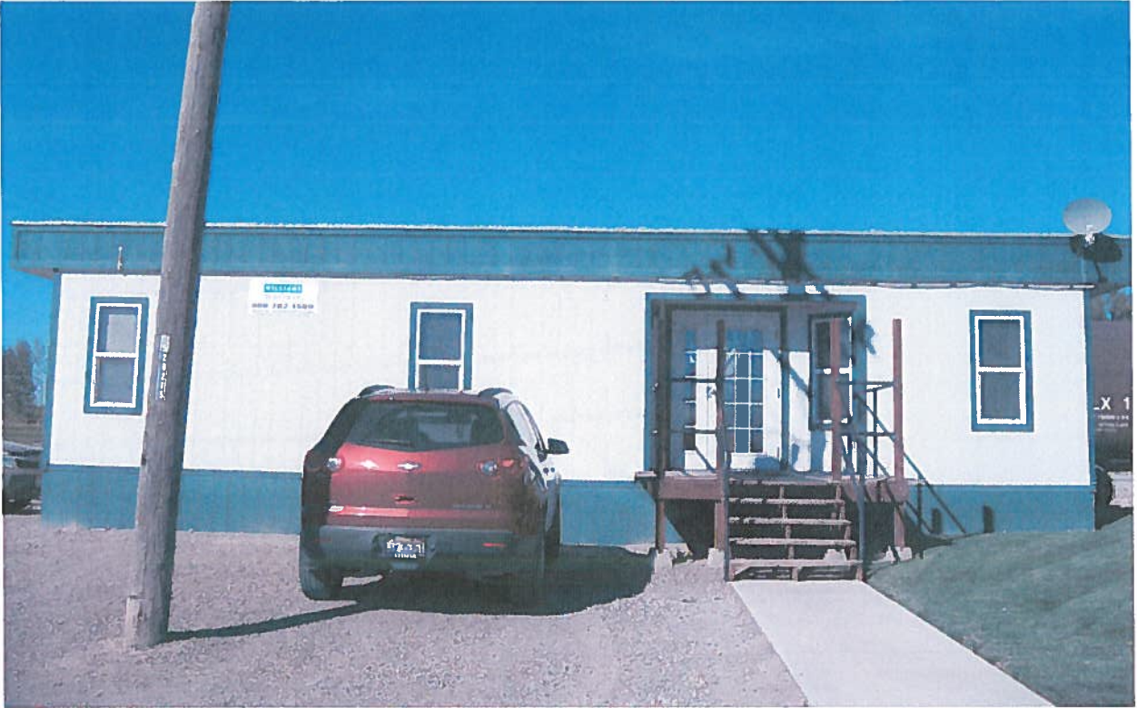
Above: Main office building with a reception desk, two private offices and a restroom
