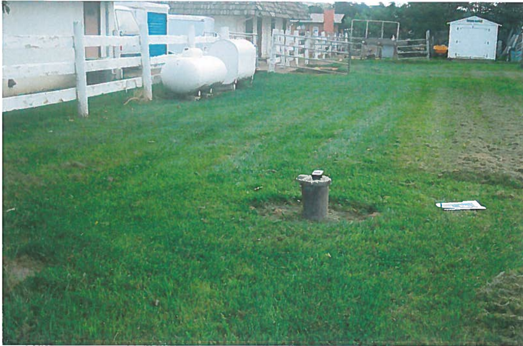
The POD – a 6 " diameter well drilled in 1987. Fitted with a Grundfos 1.5 hp submersible pump.
