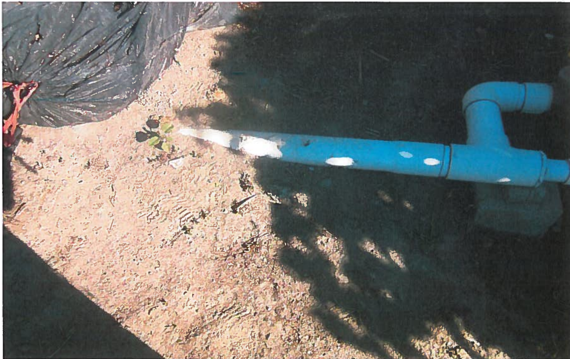
The buried 4-inch pipe for irrigation of the rest of the subdivision.
