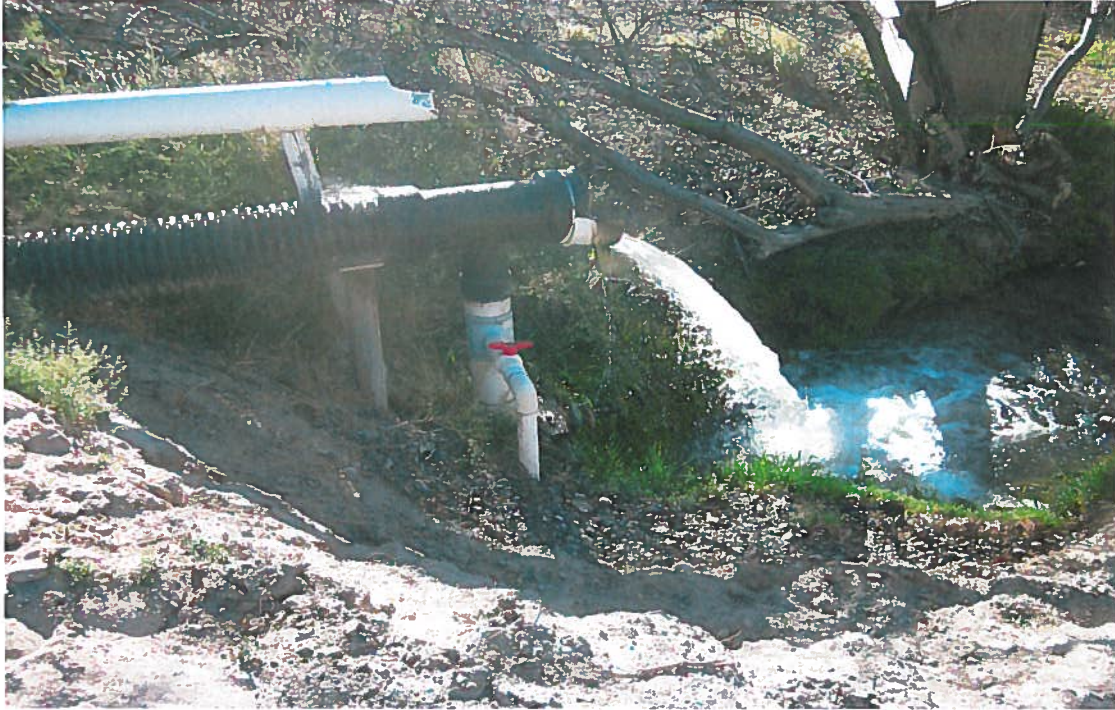
Ruby Drain water drops into lower drain ditch. There is a buried 4-inch pipe that conveys water to the pump.
