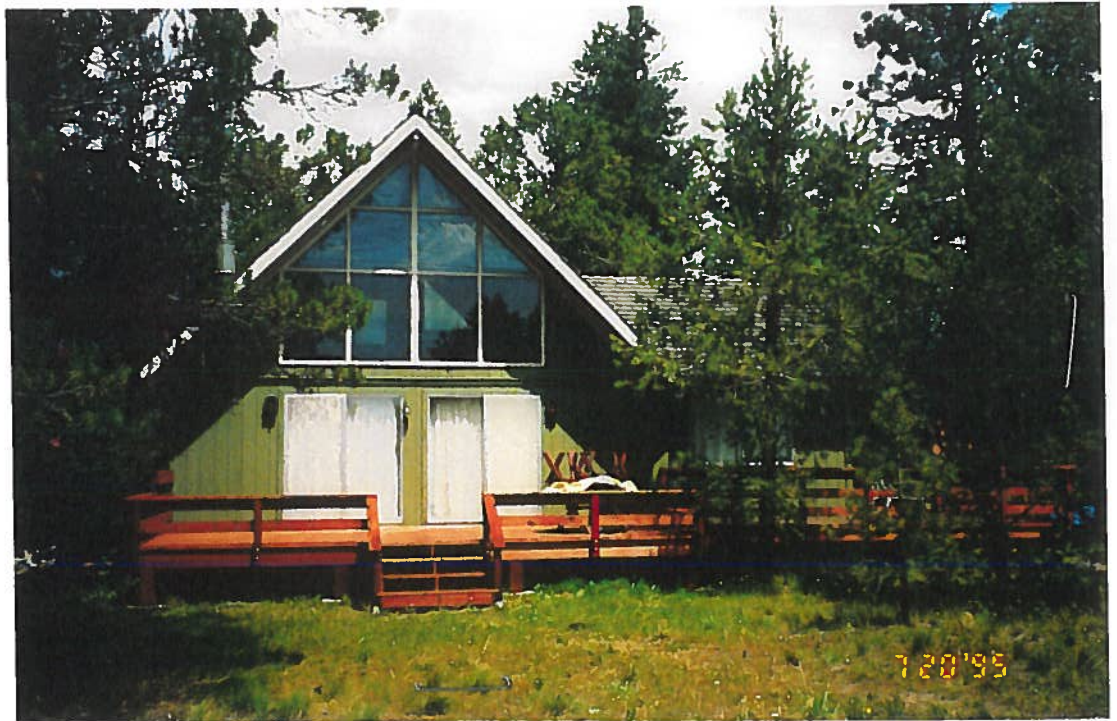
4) Typical domestic unit This one is 251 Lee Way
