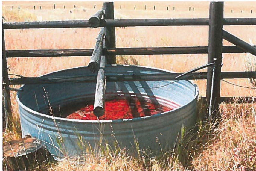
65-13890 Exam 8/14/2014: Main 1,000 gallon stock trough/tank facing west. Note pipe on left inflow from southern spring while pipe on right is inflow from northern spring. Stock trough not in use at time of photo. Photo provided by owner (Steve LaFon) during office visit 8/14/2014.
