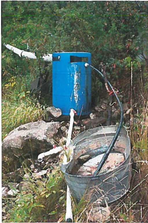
65-13890 Exam 8/14/2014: Photo on right is northern spring (main source of water year round). Plastic pipe from spring into blue barrel collection piped via 1½" pipe to stockwater troughs + faucets and ½" black poly pipe to camp trailer site. Photo on right southern spring (secondary source, spring does not run after ~ August each year). Photo provided by owner (Steve LaFon) during office visit 8/14/2014.
