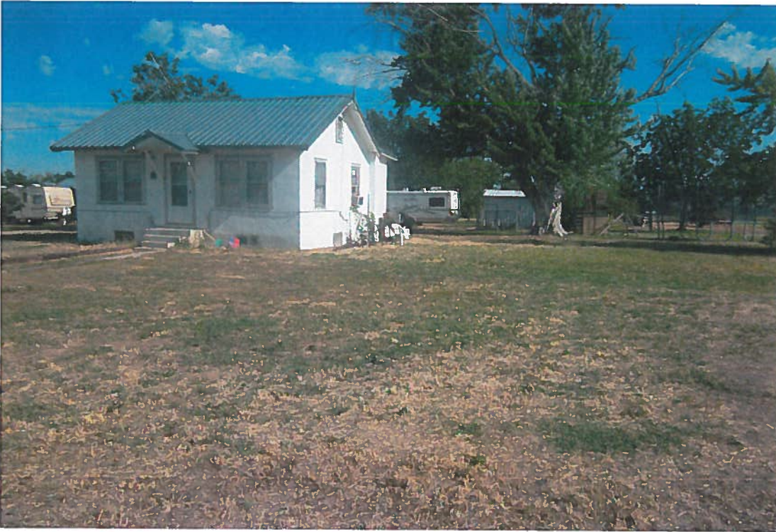
House and yard # 2. Domestic use is from an old hand dug well, water right no. 65-3262. This right will provide backup domestic. The residents irrigate from this well with a garden hose.
