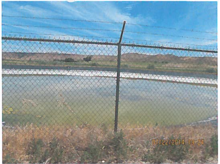
Wastewater storage pond
