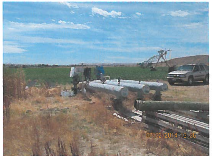
Pumps from King Hill Irrigation ditch
