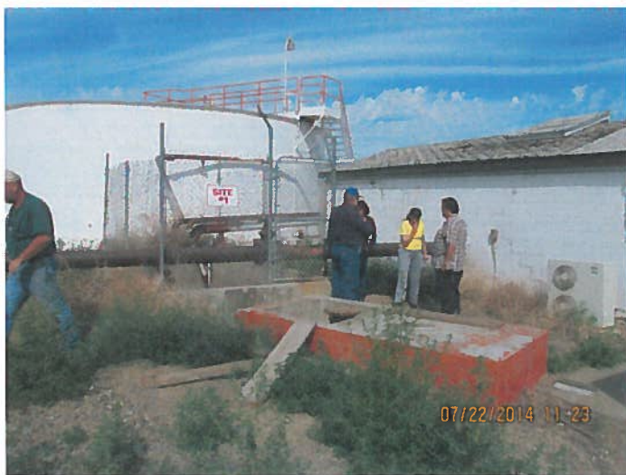
Well location in center of group and clarifier (round tank)
