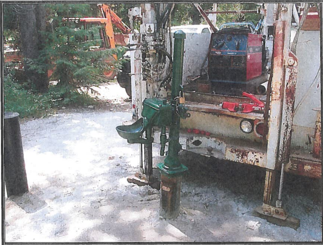
LOOKING WEST AT PARTIALLY INSTALLED NEW HAND PUMP 44.55.403 Lat. X 115.56.770 Long.
