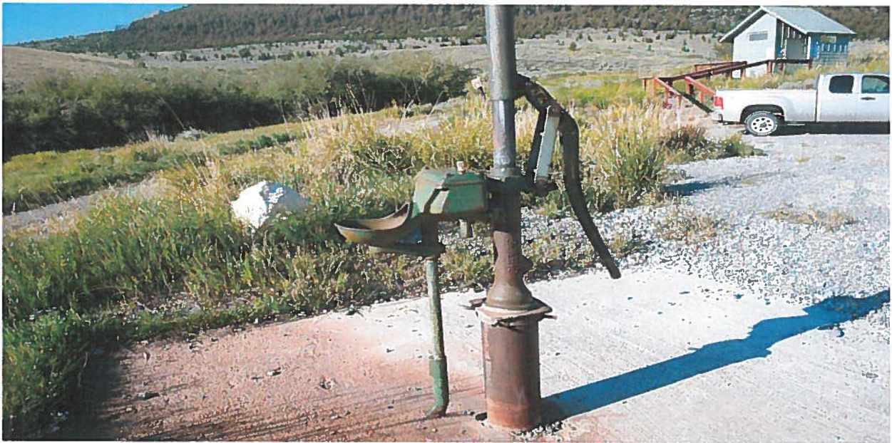
Pump at Public Site, -113.179721, 44.310379
