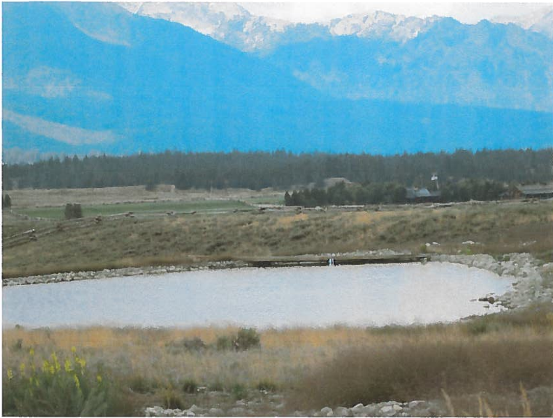
Picture 5: Pond shown with return flow stand pipe visible. Water spills into pipe and returns to the Salmon River.
