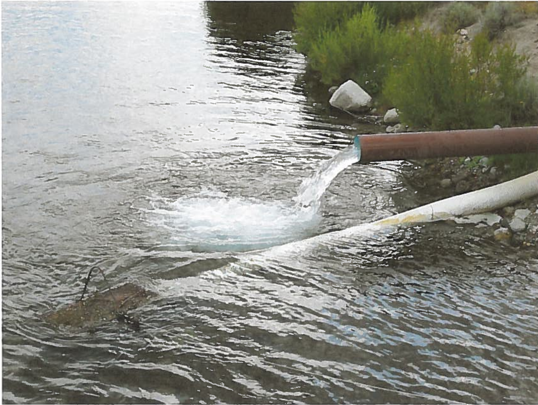
Picture 1: Point of diversion with fish screen is shown along with return flow back to the river.
