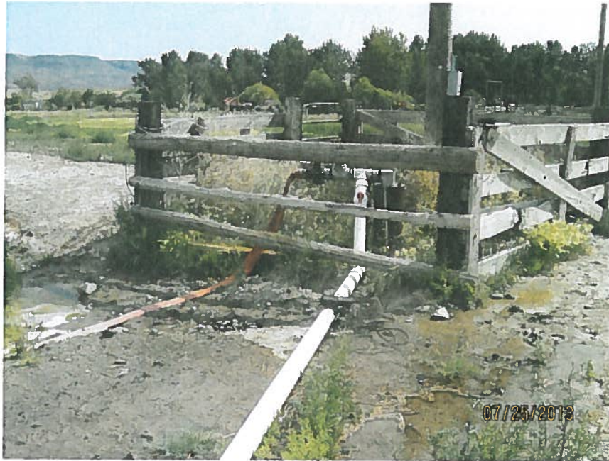
Figure 1: Well with flexible hose to pond and PVC to gated pipe.
