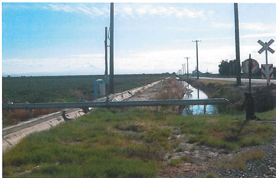
The well is a shared POD with 63-32989 and 63-32990, so, in addition to being piped underground for the supplemental irrigation of 63-11801, it can be piped into the concrete ditch and Wilder Irrigation canal, both located south of the well.
