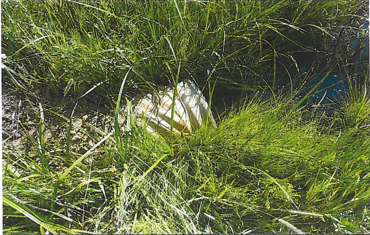
View of an 18" CMP outlet pipe located at the southeast corner of the wildlife storage pond.
