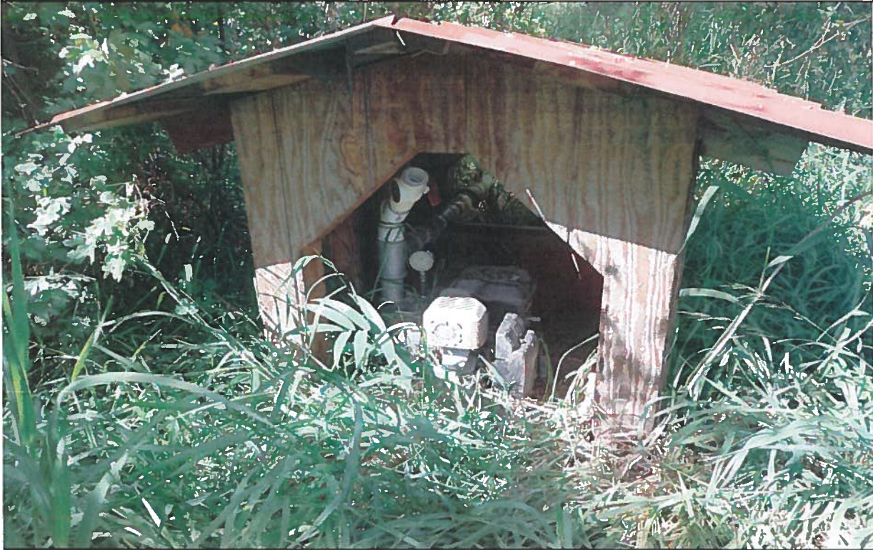
View of 5.5 horsepower gas operated pump and motor in small enclosure near the Middle Fork of the Payette River.
