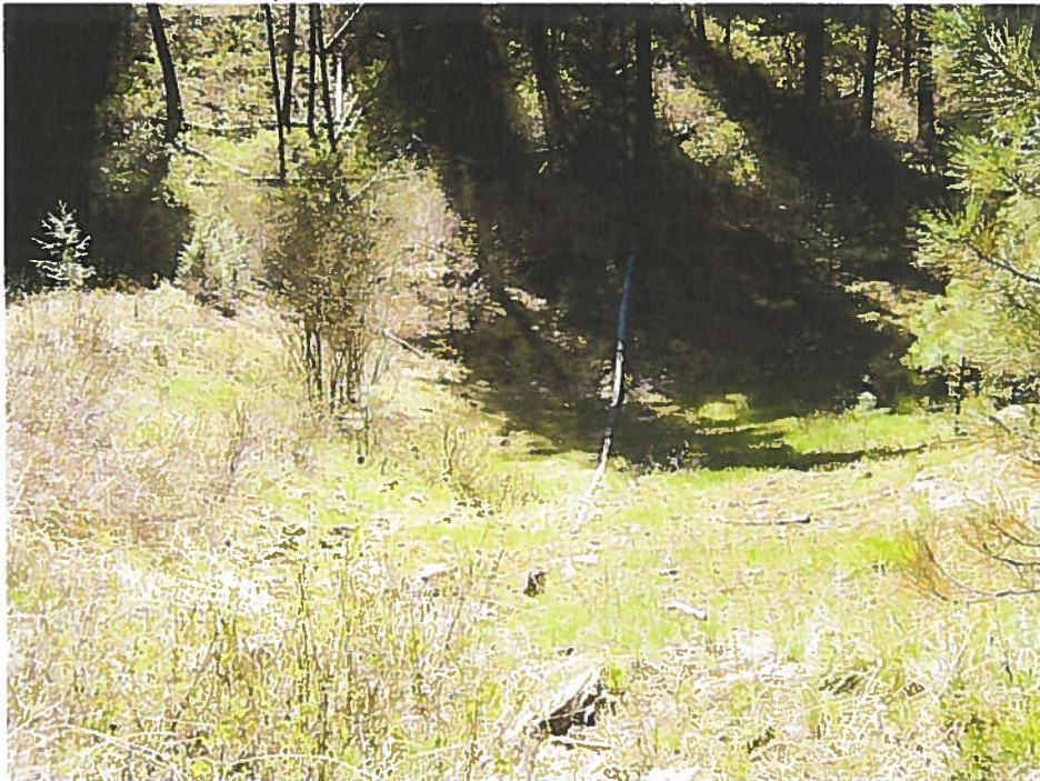
View of pond standing at the side. Dam is shown on the left side of the photo. Inlet is on the right side of the photo.
