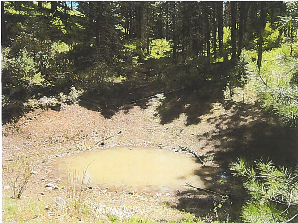
View of pond standing on dam.
