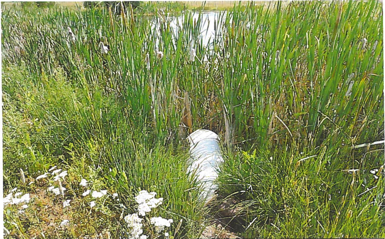
View northeasterly of the 15" PVC outlet pipe located at the south end of the wildlife storage pond.
