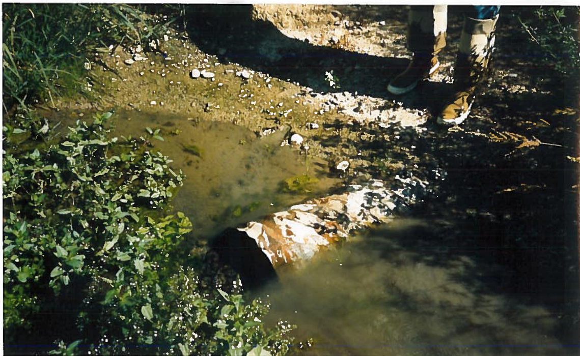
PHOTO FOUR- Taken looking northwest at a 15" culvert that is used as a means of conveyance for the water from the spring.
