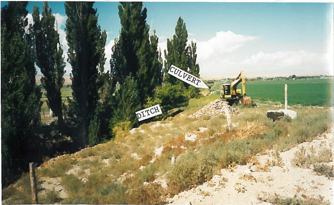
PHOTO TWO- Taken looking west towards the place where the culvert from the spring enters the drain ditch from the Buckaroo Canal.
