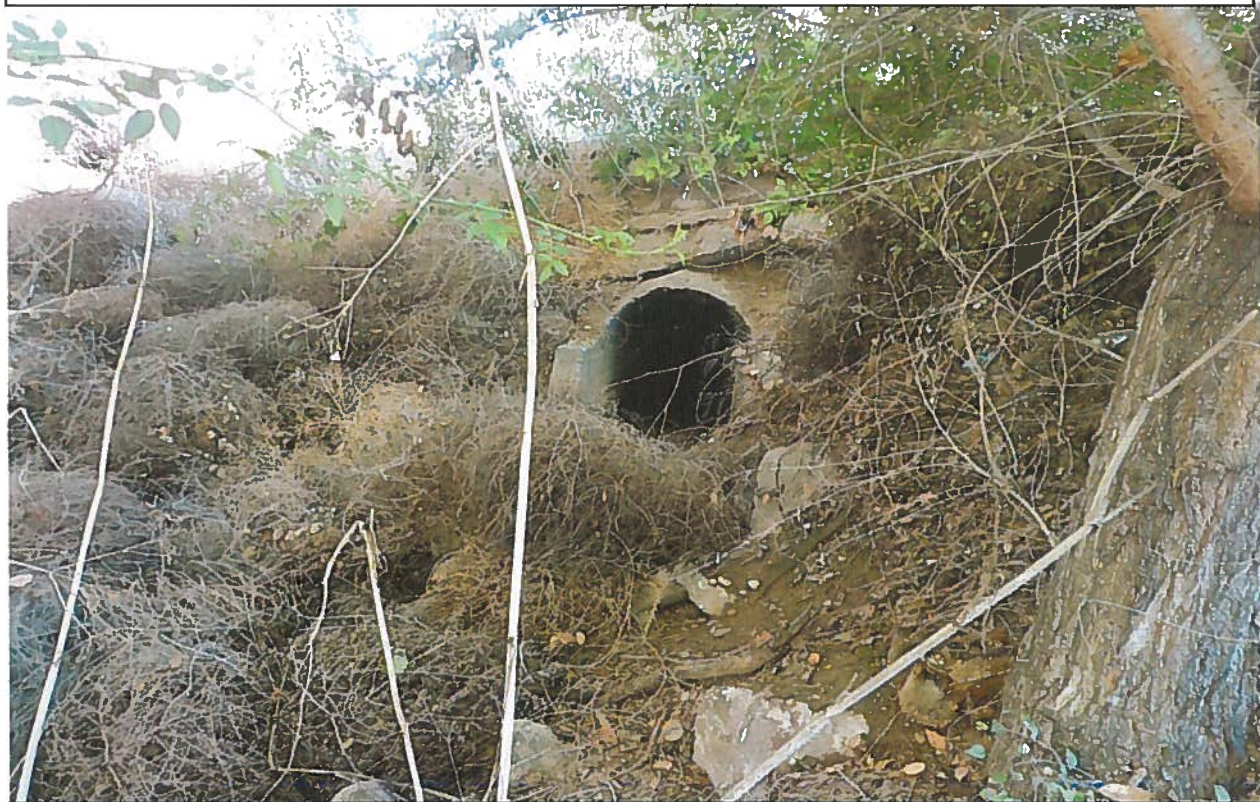
Photo 11 – View easterly of the 36" concrete arched tunnel/culvert at Frost Lane.
