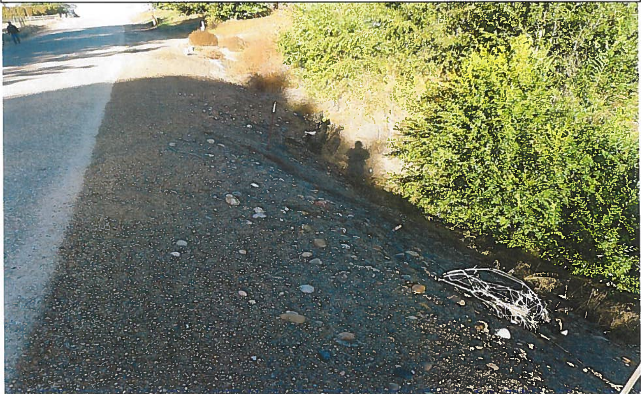
Photo 9 – View westerly of the road embankment over the Escott Drain. The top of the roadway embankment is approximately 10' above the top of the 36" diameter concrete tunnel/culvert.
