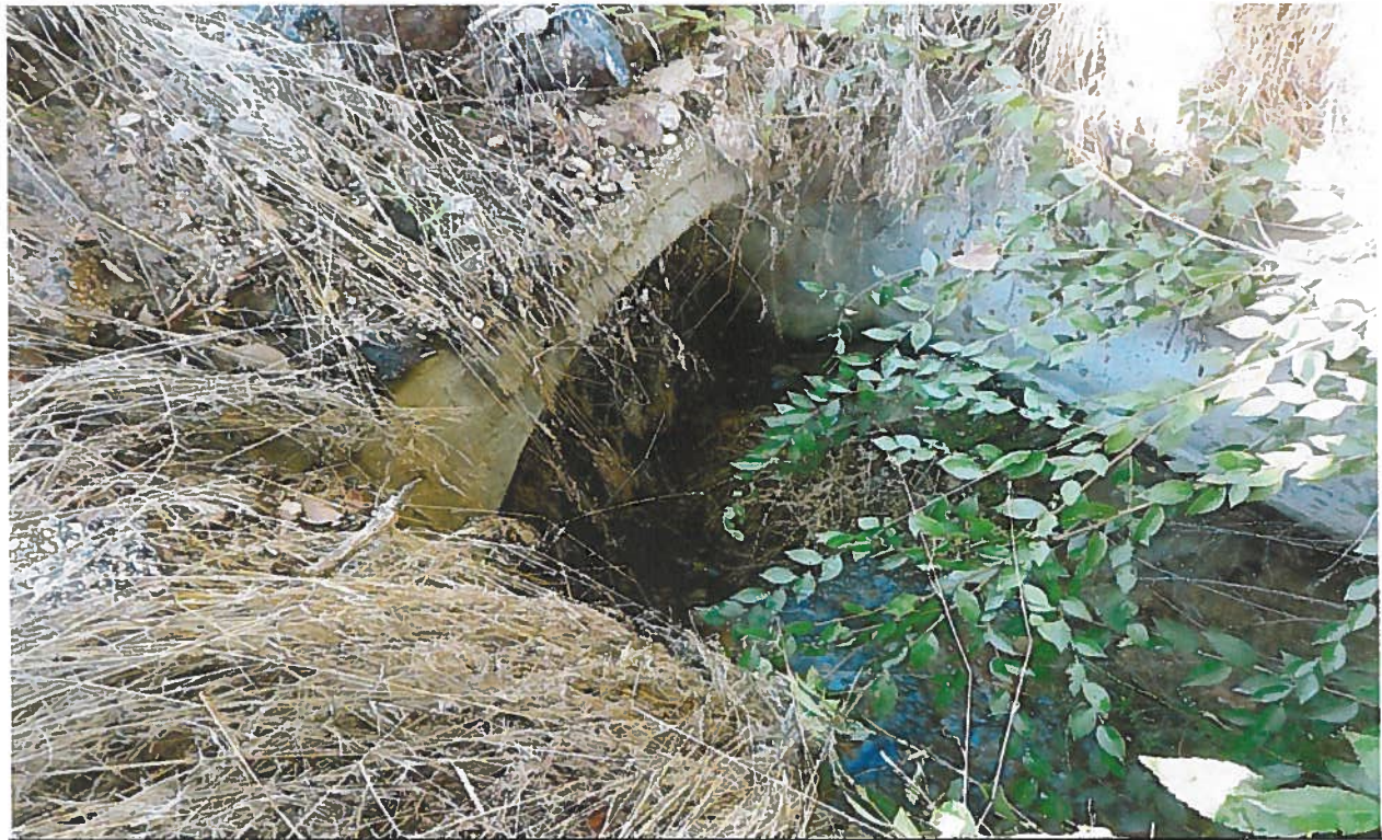
Photo 8 – View of the 36" diameter arched concrete tunnel/culvert beneath Pear Lane.
