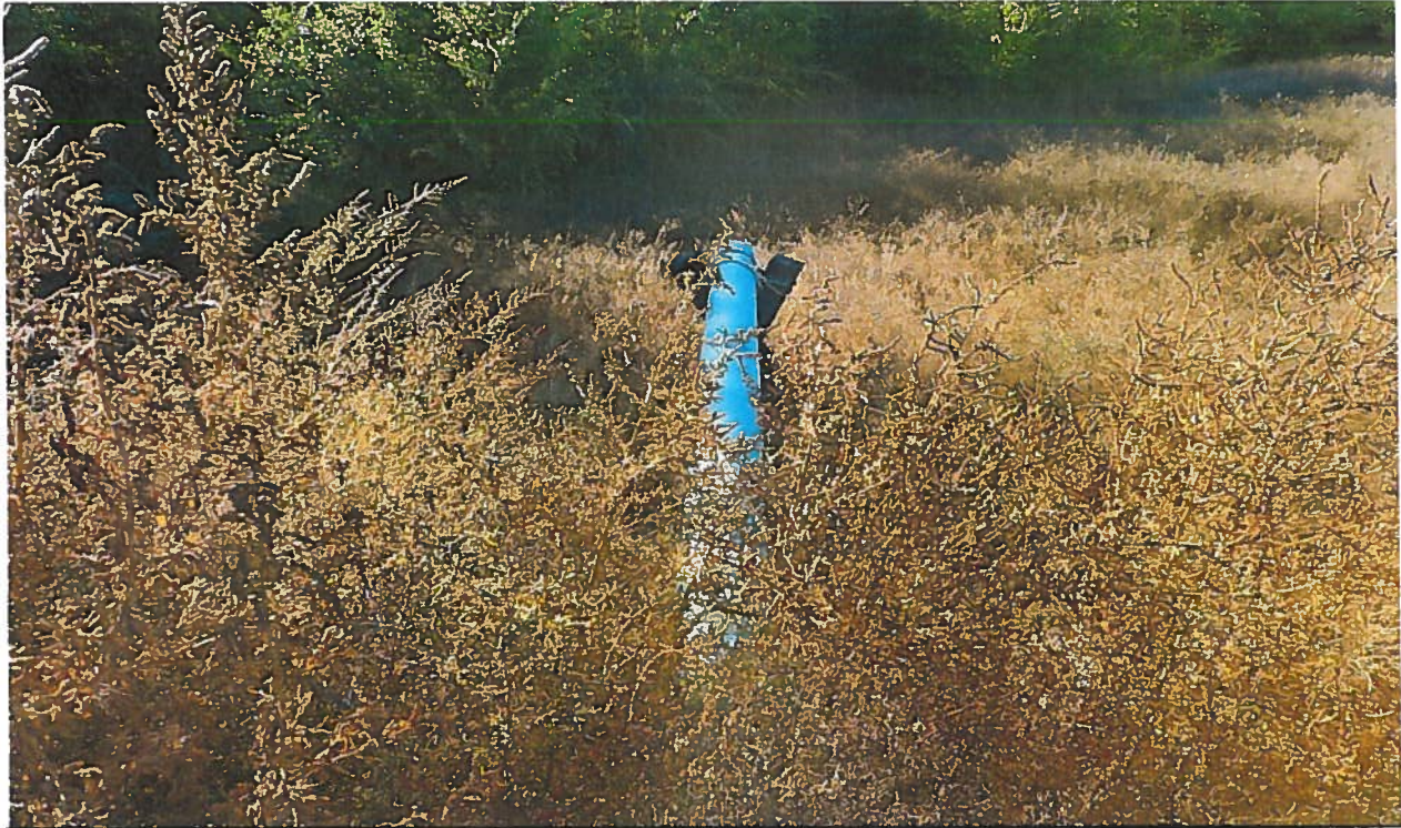
Photo 6 – View southerly of the west 12" PVC overflow pipe. Overflow water from the storage pond will discharge onto the downstream slope of the dam.
