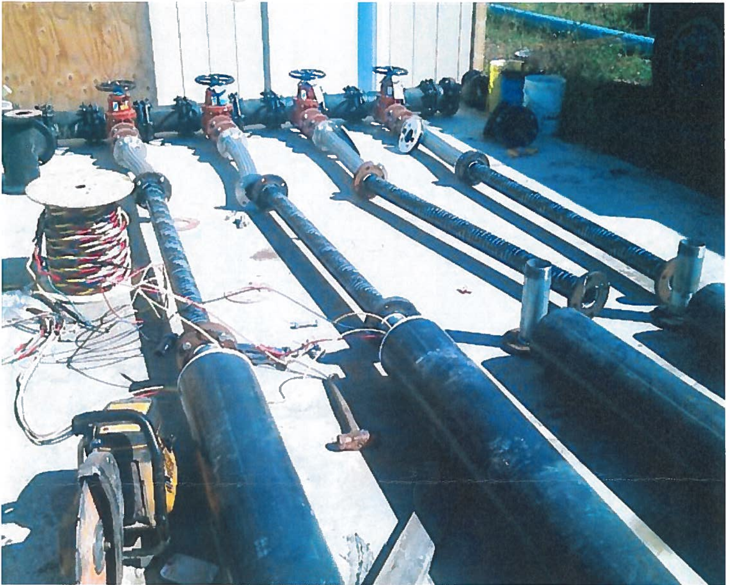
Raw Water Intake Pump Manifold Extension Under Construction (2008)
