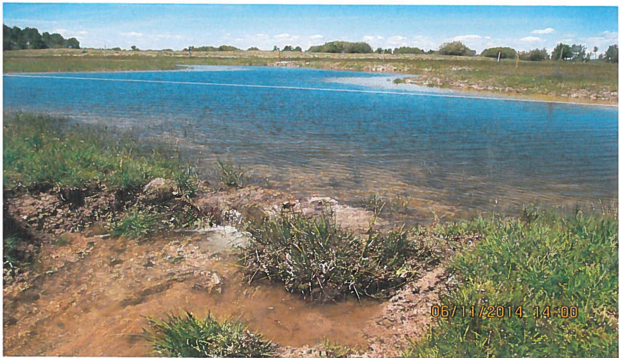
Pond # 2 outlet, looking North
