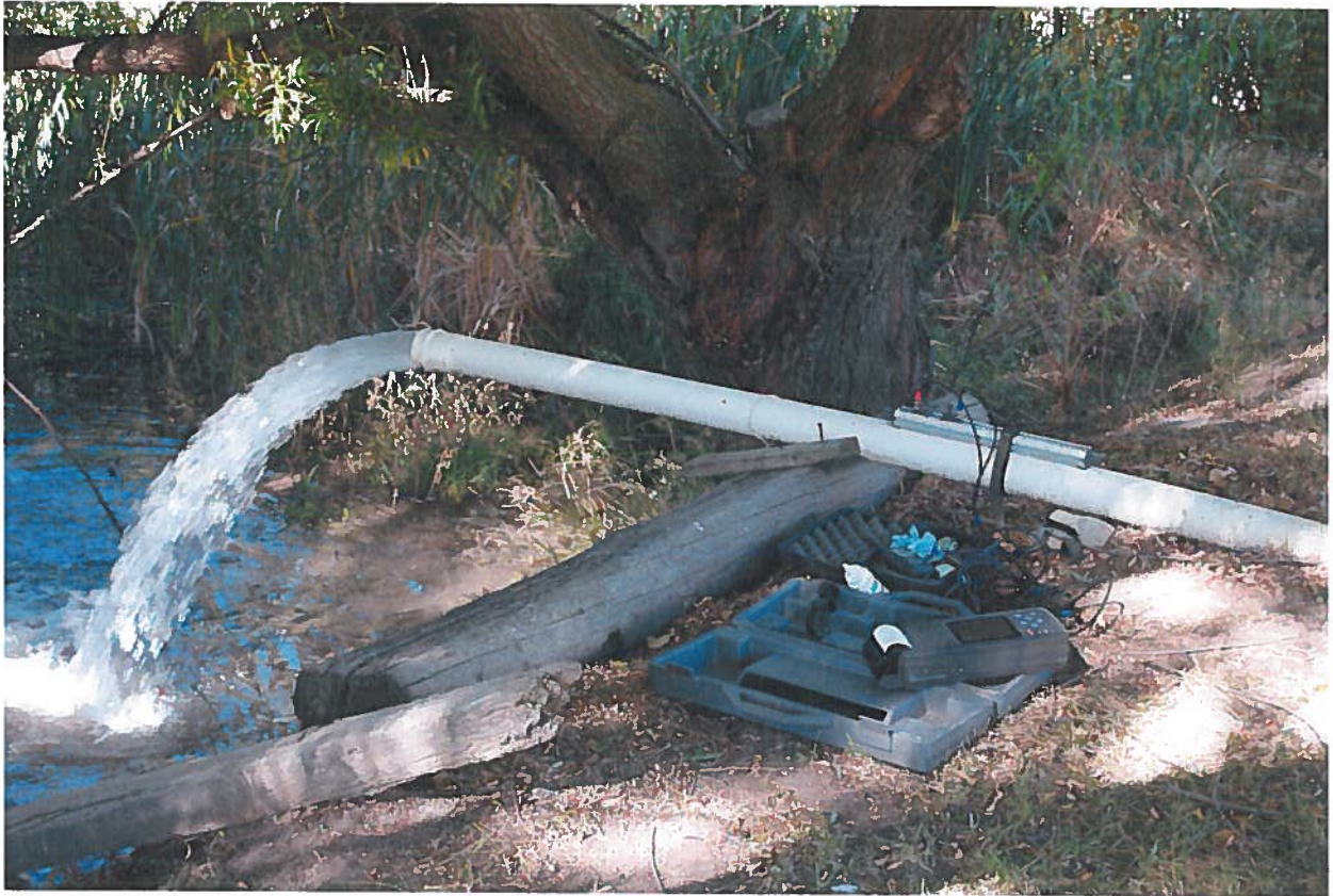
Outlet to Pond 1
