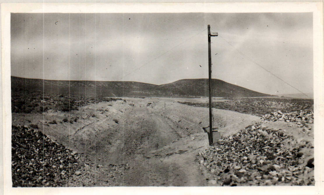
Canal A, high line from Plant No. 1.
