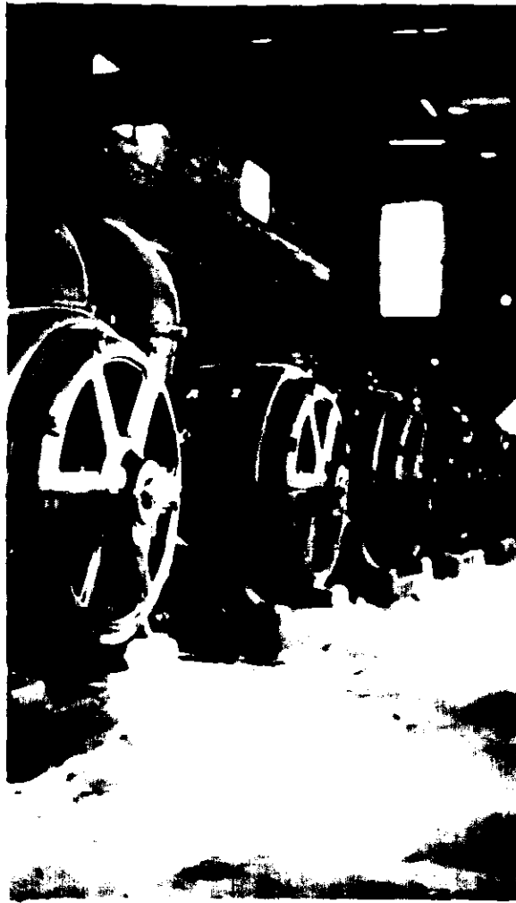
Interior of Pumping Plant No. 1.
