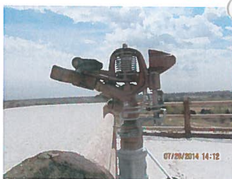
The riding arena (left) is irrigated with Aqualink Impact Rotor sprinklers (center). It also has one automatic horse watering station (right).
