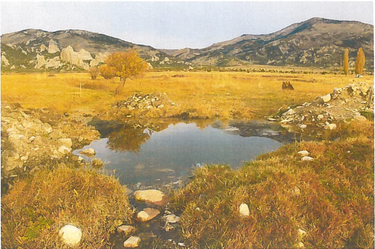
Test pit for pond – November 6, 2014
