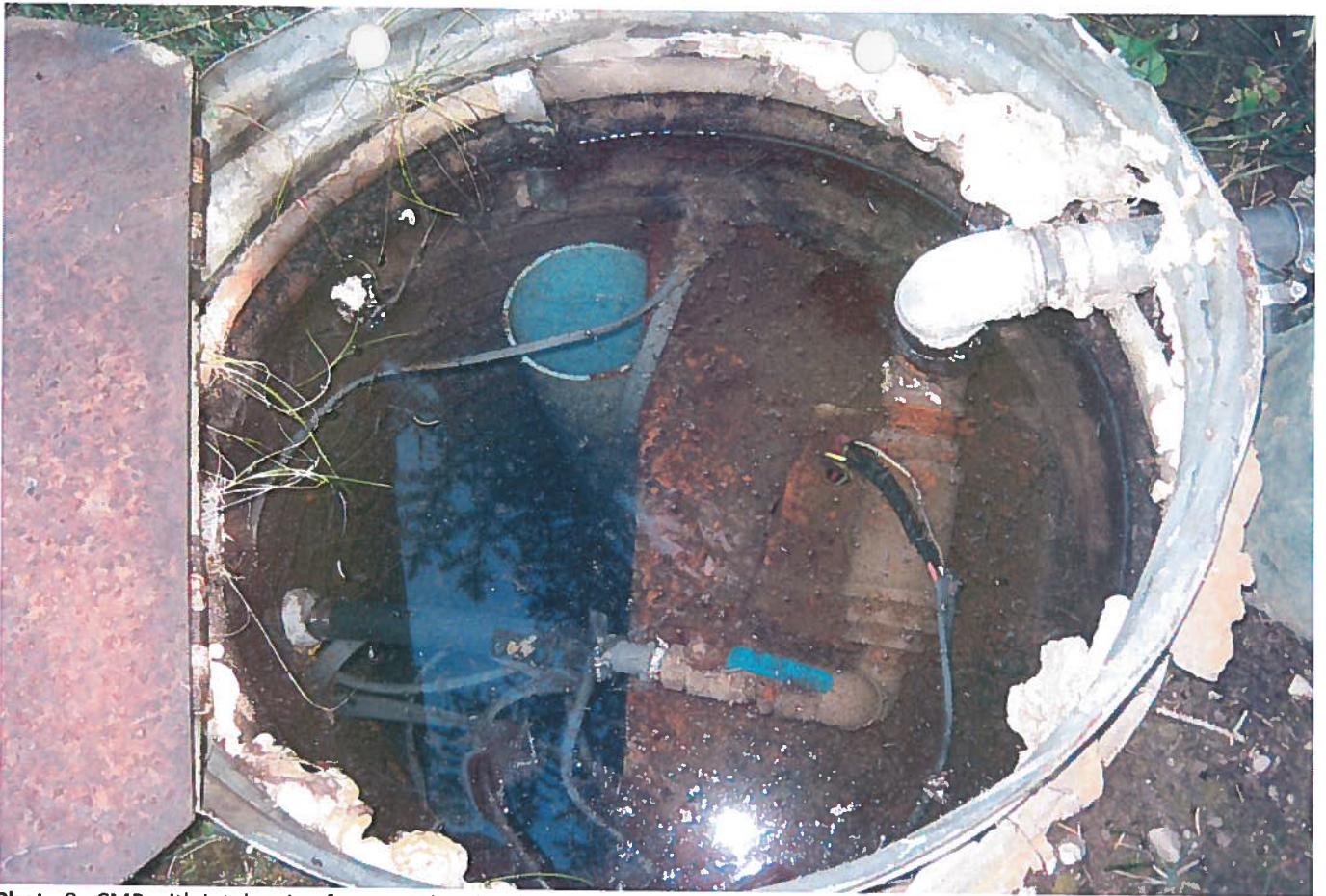
Photo 9: CMP with intake pipe from pond with valve and small irrigation pump/discharge pipe to sprinkler system.
