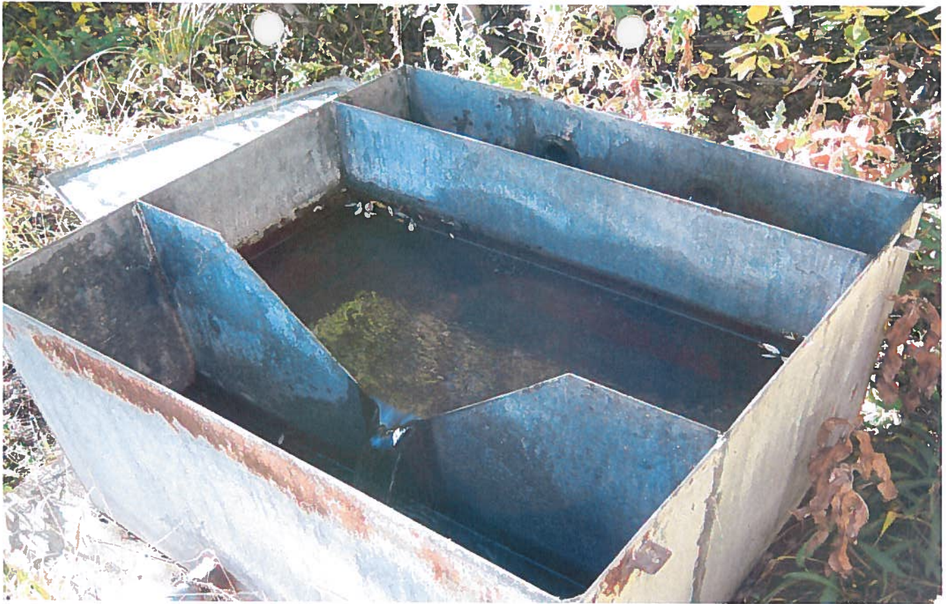
Photo 1: Weir box with baffle and 90° V-notch weir. Inflow to box from spring source/diversion.
