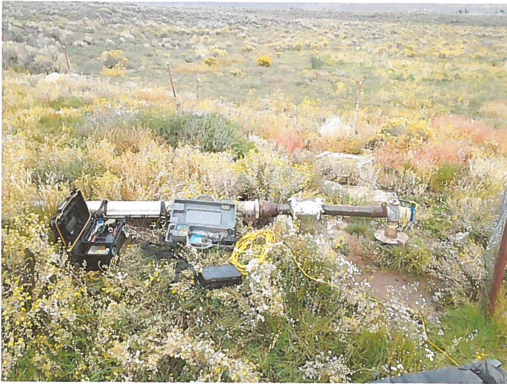
Verification of flow using ultrasonic meter
