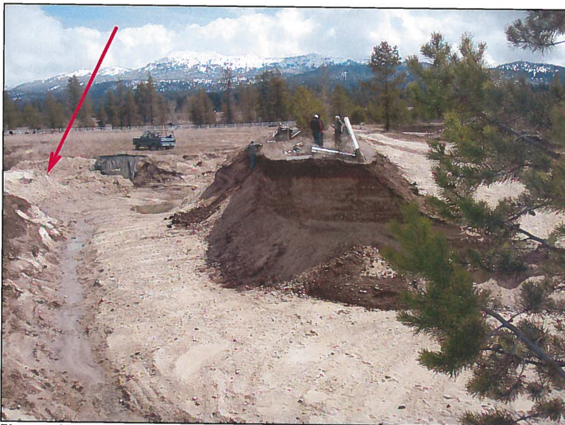
Photo 3 - View is looking east along the approximate south line of the Baldwin's property. Shown left is the new barrier; on the right (out of view) is the neighbor's active quarry.
