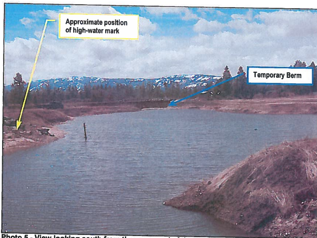
Photo 5 - View looking south from the upper end of the pond. Note the approximate high water mark created by the previous reservoir. In the background is the location of the temporary berm shown in the photos above.
