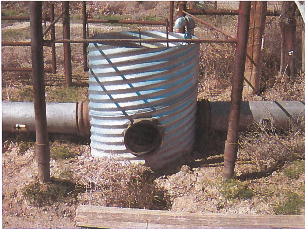
Figure 2: Diversion culvert where discharge was measured with Sparling Meter.
