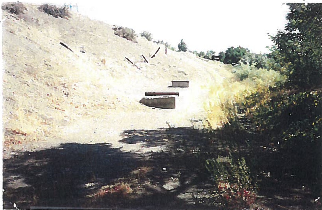
Access ports to infiltration gallery.
