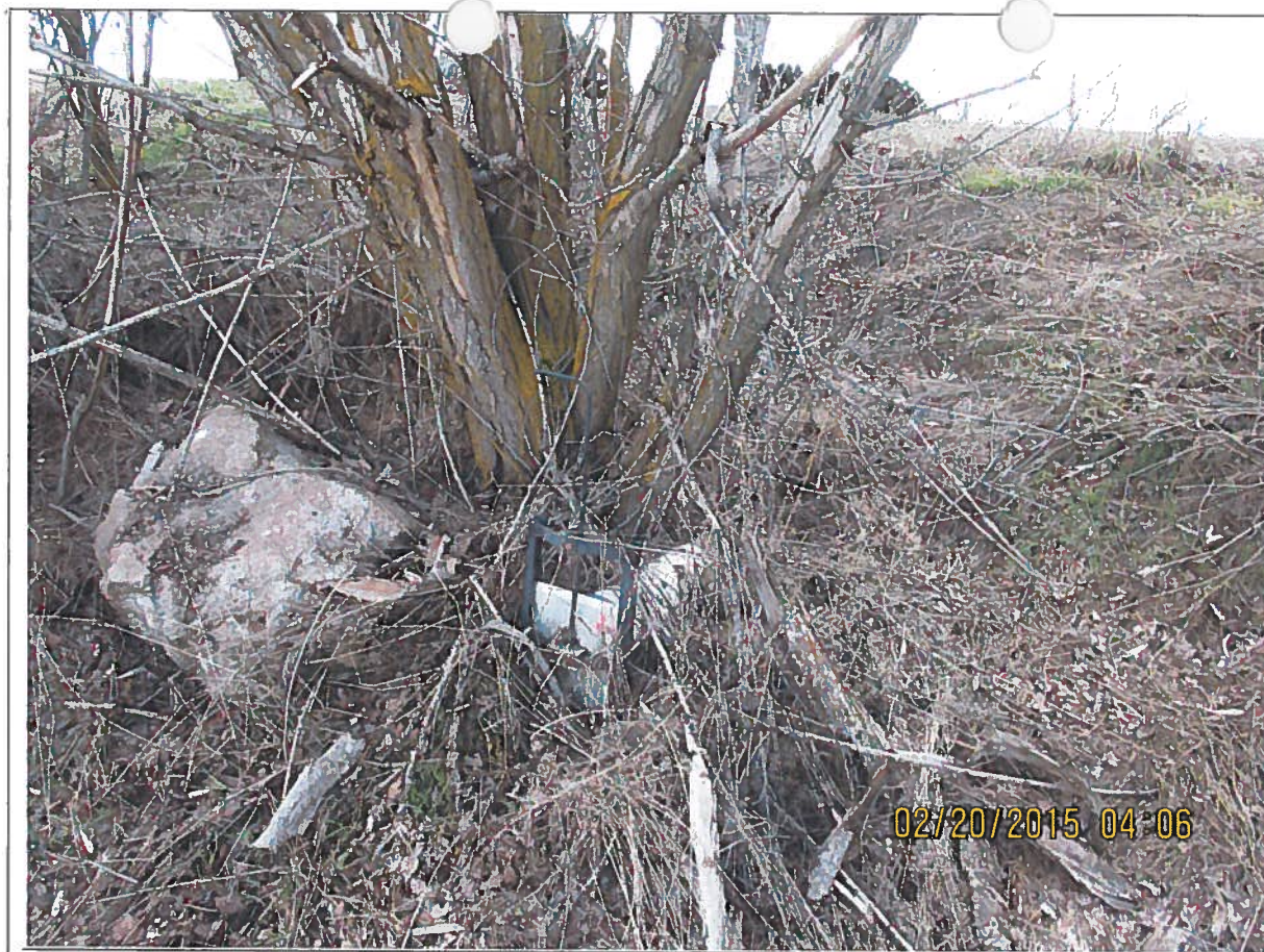
Outlet in SW corner of pond.
