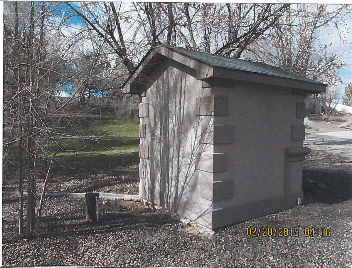
Point of Diversion located near driveway on east side of property.
