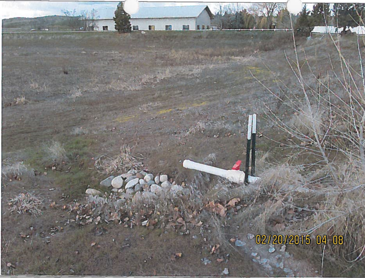
Inlet to pond located on east end of pond.
