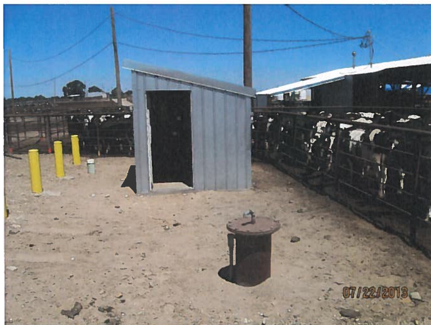
Figure 3: Well #2 (D0025278) and pump house.
