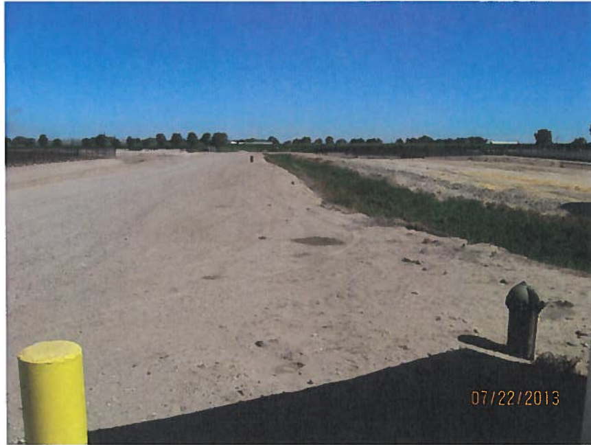
Figure 5: Well #3 (D0046509) is in right foreground and Well #8 (D0048277) is in background along south (left) side of drain ditch.
