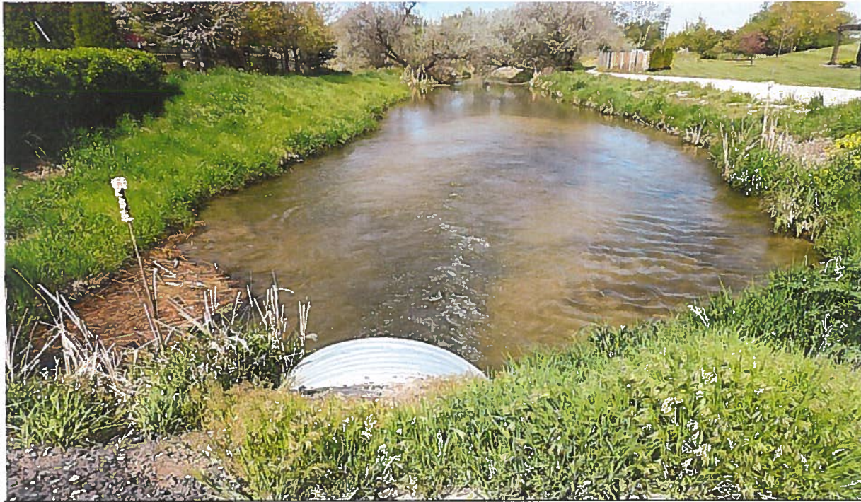
View westerly of the 60" CMP discharge pipe from the HOA aesthetic storage pond. The waterway continues northwesterly through the Banbury Meadows development and Banbury Golf Course prior to discharging to the Boise River.
