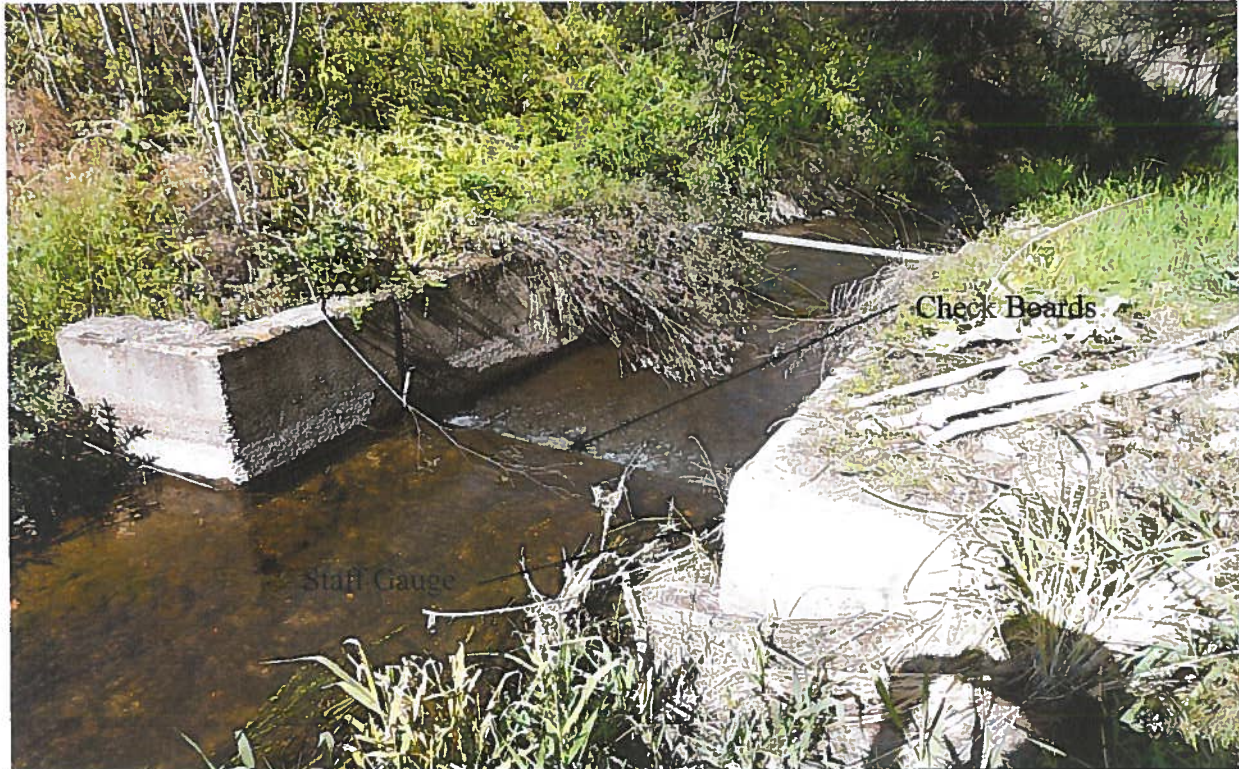
View southwesterly of a concrete flow measuring structure in Warm Springs Creek. The structure is approximately 100' downstream from the 36" CMP discharge pipe from the Boise River. A staff gauge is mounted to the northerly abutment upstream of the flow control boards.
