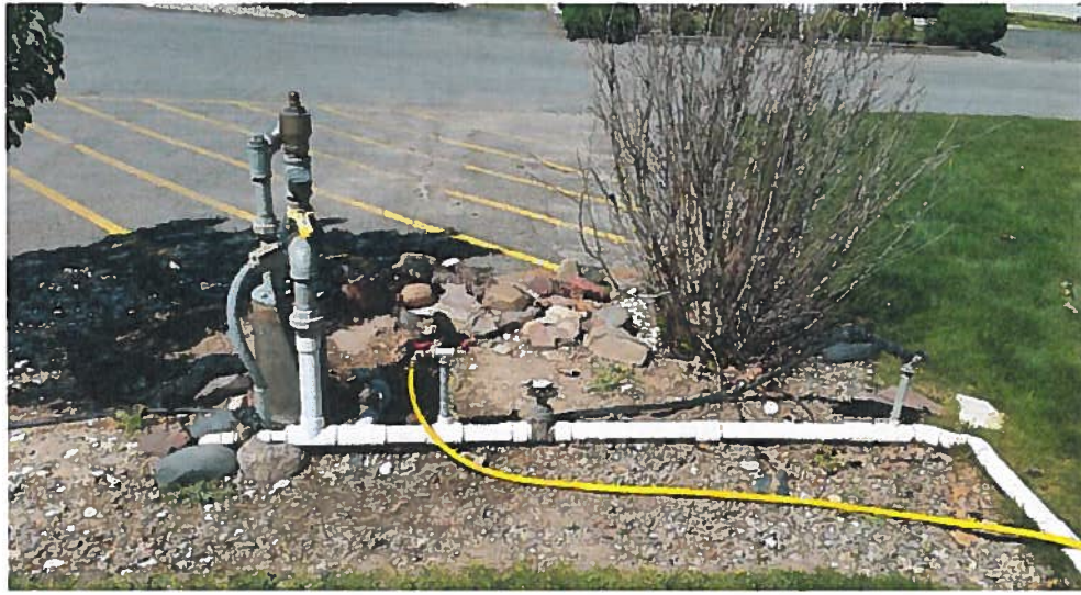
Figure 1: NENE well facing northerly. Ground water from the NENE well is discharged into an above ground 2-inch Sch. 40 pvc manifold that is used to direct the well water to three separate irrigation zones: (1) an underground 1-1/4 inch pvc mainline feeding a 6 zone underground sprinkler system for the clubhouse and common area (west/left branch in photo), (2) a 2-inch above ground pvc mainline with 1/2-inch risers and spigots for each of the 32 home lots in the northern central block (east/right branch in photo), and (3) a 2-inch above ground pvc mainline with 1/2-inch risers and spigots for each of the 26 home lots in the outer northeast block (north branch/straight branch in photo).
