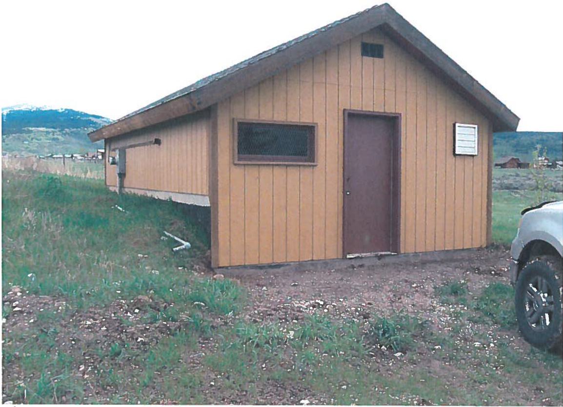
"New well" pump house
