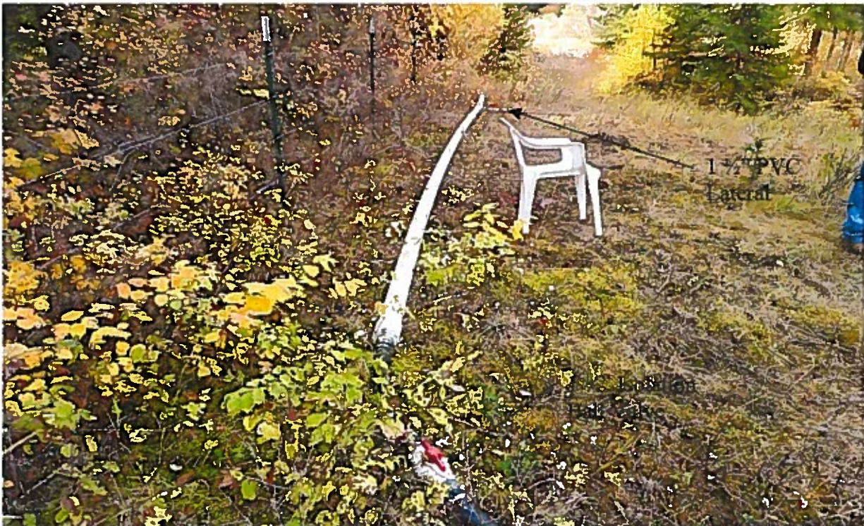
View westerly of the 3" PVC supply line where the supply line is reduced to 1 1/2" PVC. A 1 1/2" isolation ball valve is installed to isolate the 1 1/2" PVC supply line. The 1 1/2" PVC supply line terminates at a frost free hydrant near the right holder's home.
