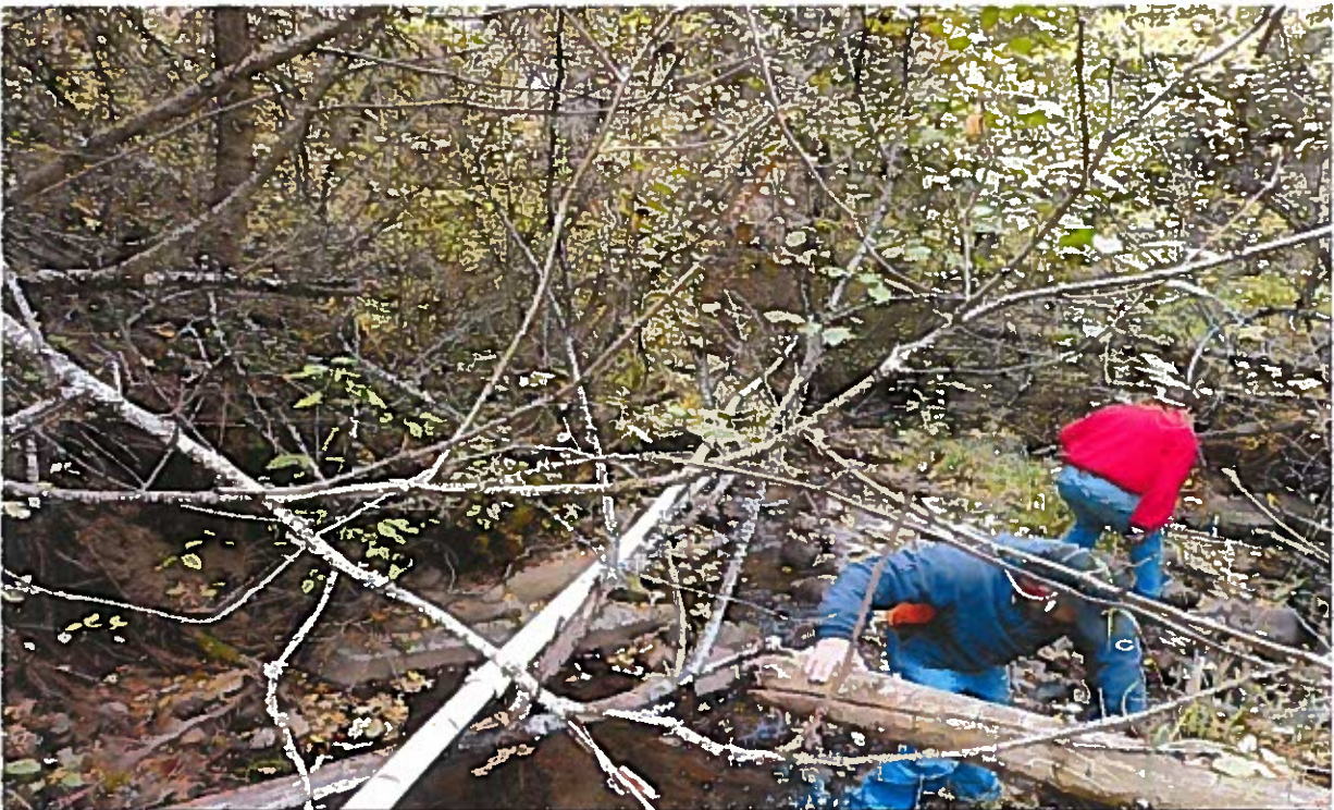
View easterly of the 3" PVC supply line from Trail Creek.
